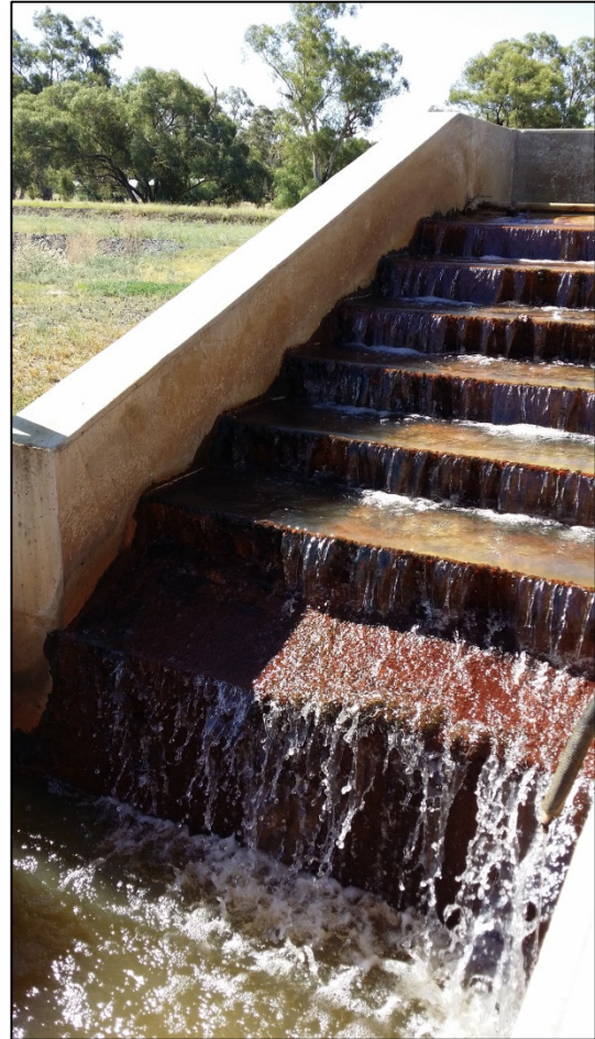
Figure 4-2: Step Aerator (in Operation)
