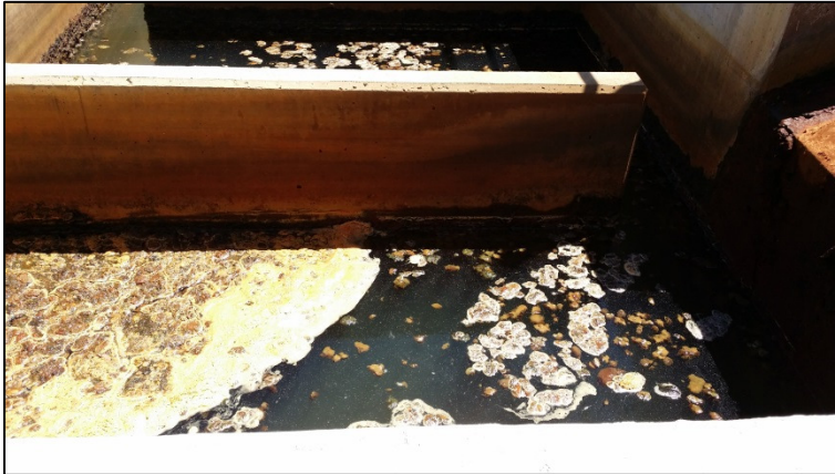
Figure 4-5: Algae in Flocculation Chamber
